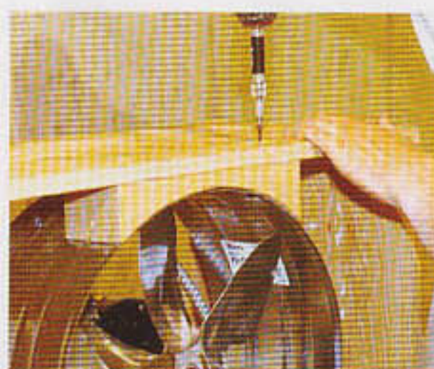
11 Screw the blocks flush with the rear face of the ply box so they hold the fan in place
