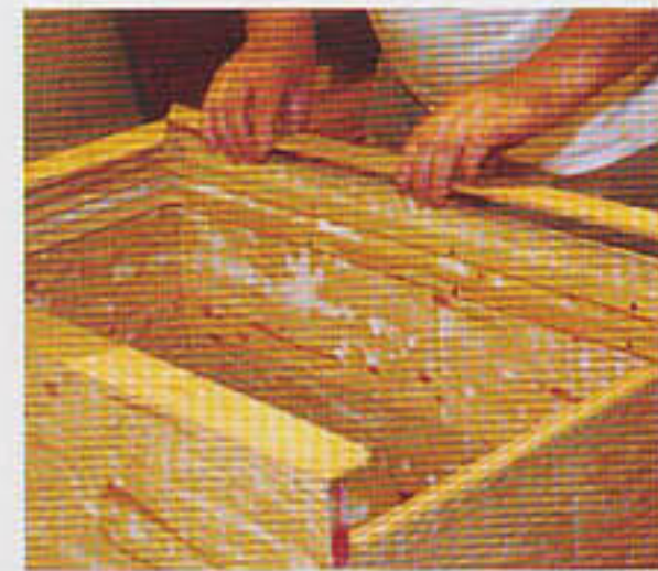
08 Glue and screw 6mm to the front to act as a holder for the primary filter and prevent it falling out. Sand the edges
