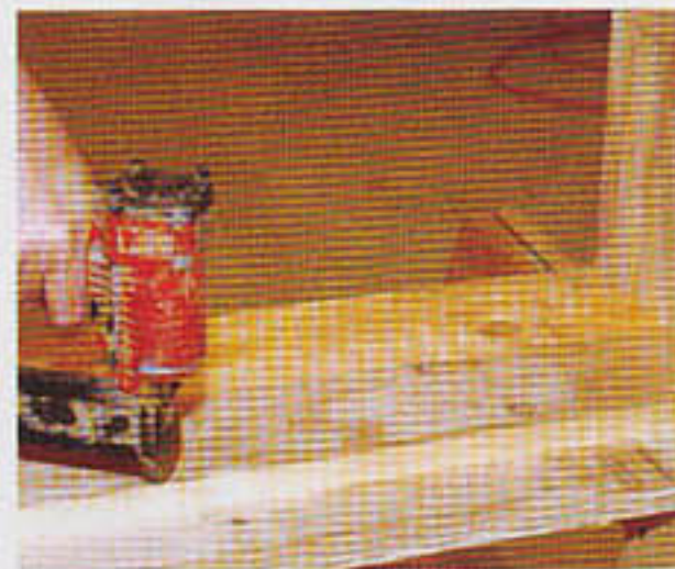
07 Glue and pin on the filter battens, making sure that they are parallel with the front edge of the box
